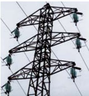
63 kV RTE, France
